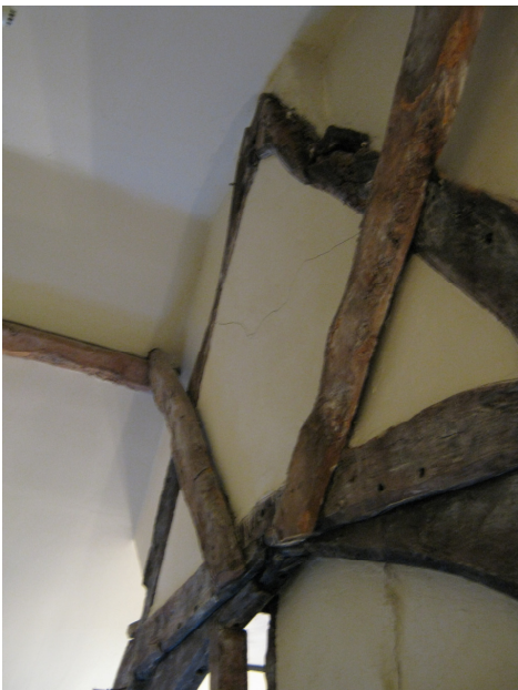
Section of interior crucks dated to 1350
